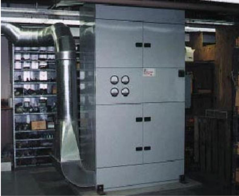
when a valve was being degassed. Before a valve can be put into service, it must undergo extensive decontamination which can last from four to eight weeks. The special media formulation labelled MM-8000 had to be designed to absorb high concentrations of mercuric compounds for these periods and relatively low trace amounts during times when degassing was not occurring.
