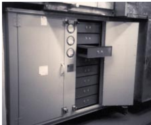
Typical USAH-404 filtration unit.
